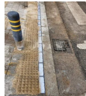
Filling the gaps with silica sand
