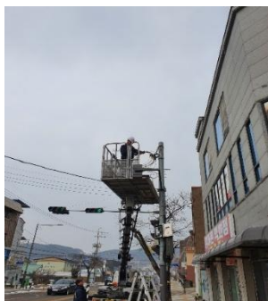
Power supply line connection
