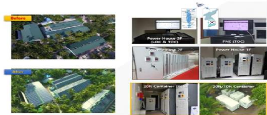
PV 300kW + ESS 1.3MWh (Micro Grid project in Maldives Resort : TOC 1))
